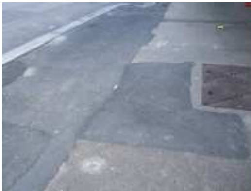
Uneven patchy bitumen surface
